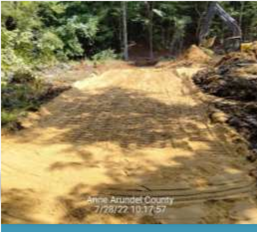
Placement and Compaction of Sand
