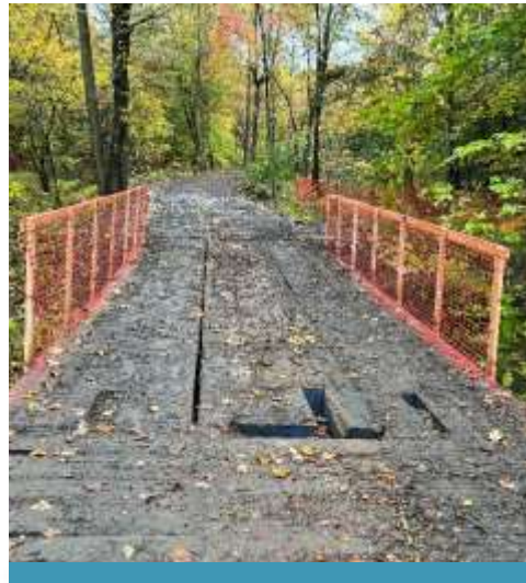
Timber Mat Bridge
