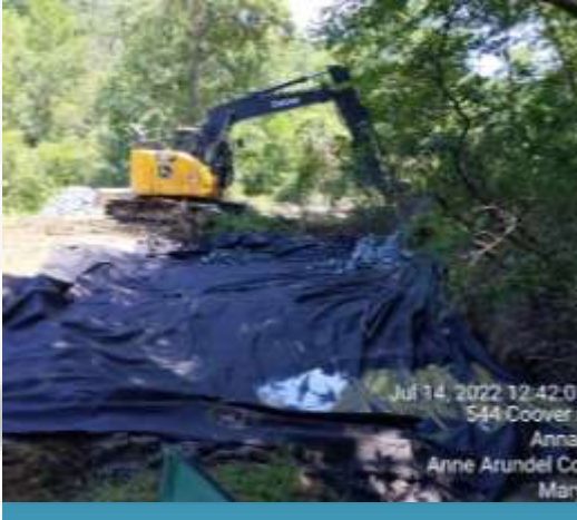
Installation of stone, riprap and geotextile
