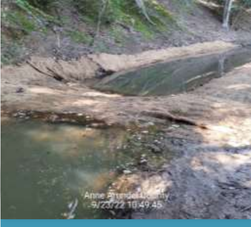
Placement of compost and soil stabilization matting
