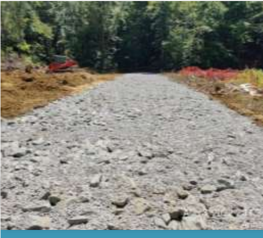
Placement of stone and gravel veneer
