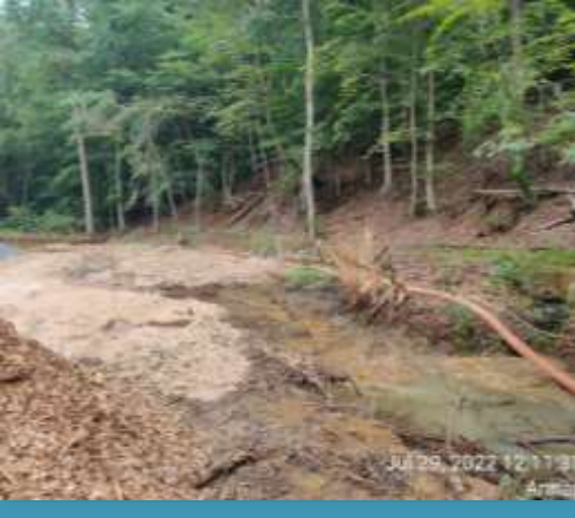
Excavation for Clay Channel Block core.
