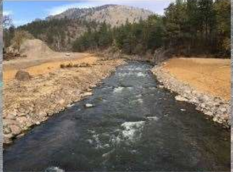
CONSTRUCTED RIFPLE WITH BOULDER VANES (TYP.)
